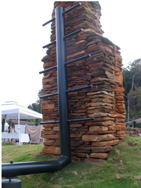
Summer 2010: Chimney with permanent preservation structure
