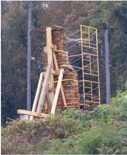
Fall 2009: Protective scaffolding for the chimney
